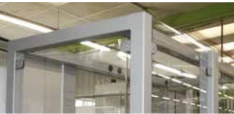
Application of PC panel support clamps
